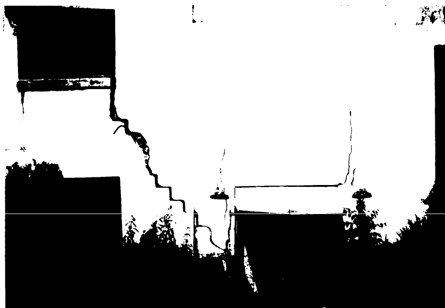
b. Diagonal and vertical cracks
